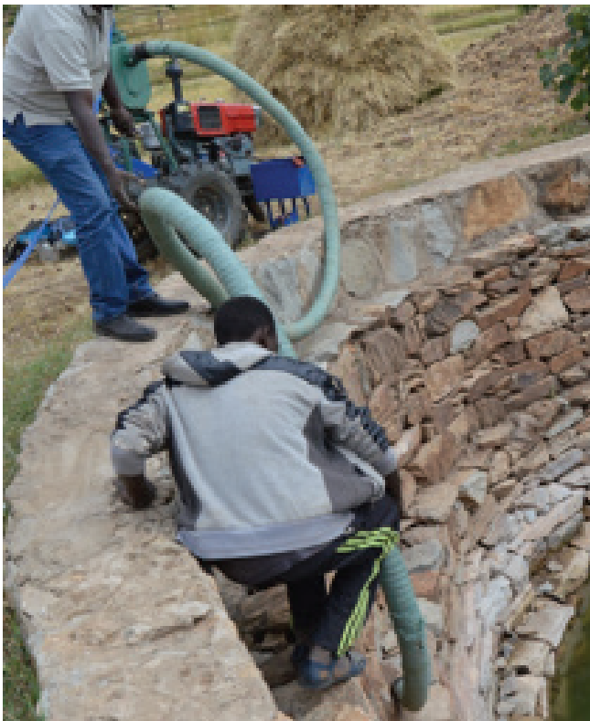
Fig 95 & 96. Inserting the suction pipe into the well (water point).
