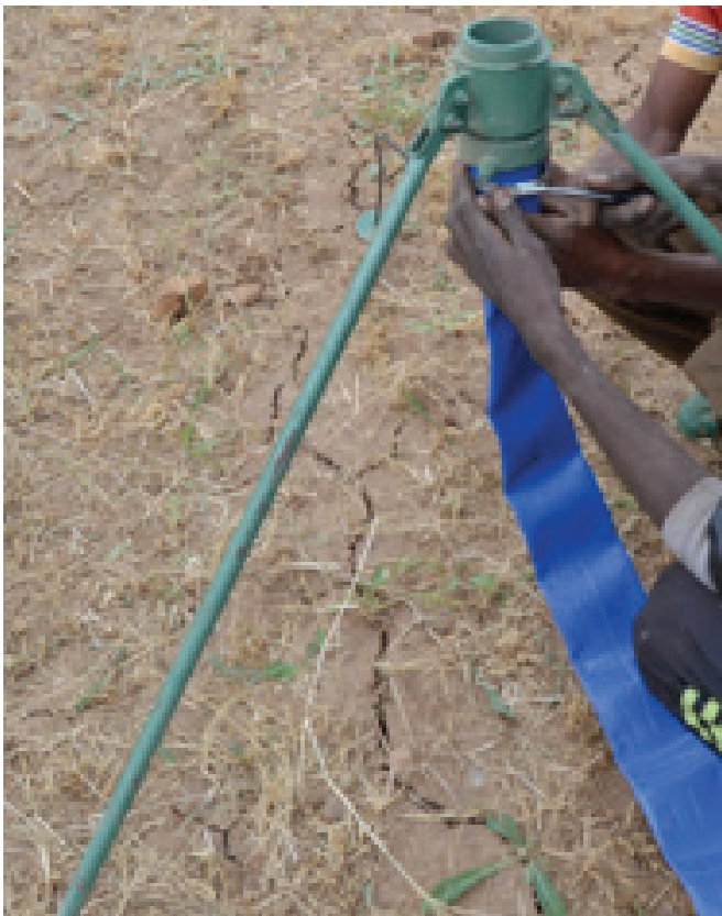
Fig 92. Inserting the discharge pipe at the center of the tripod and tighten the clamp properly with a screwdriver.
